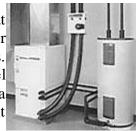
Ground source heat pumps work by circulating water or a water/antifreeze solution through a closed loop of polyethylene pipe that is buried in the ground or set beneath the water. GSHP systems can be lad out in different orientations, depending on the situation. A closed loop system, the most popular, can be laid out either vertically in 50 -250 foot deep holes drilled like a well, or horizontally in 3-6 foot deep trenches. The
